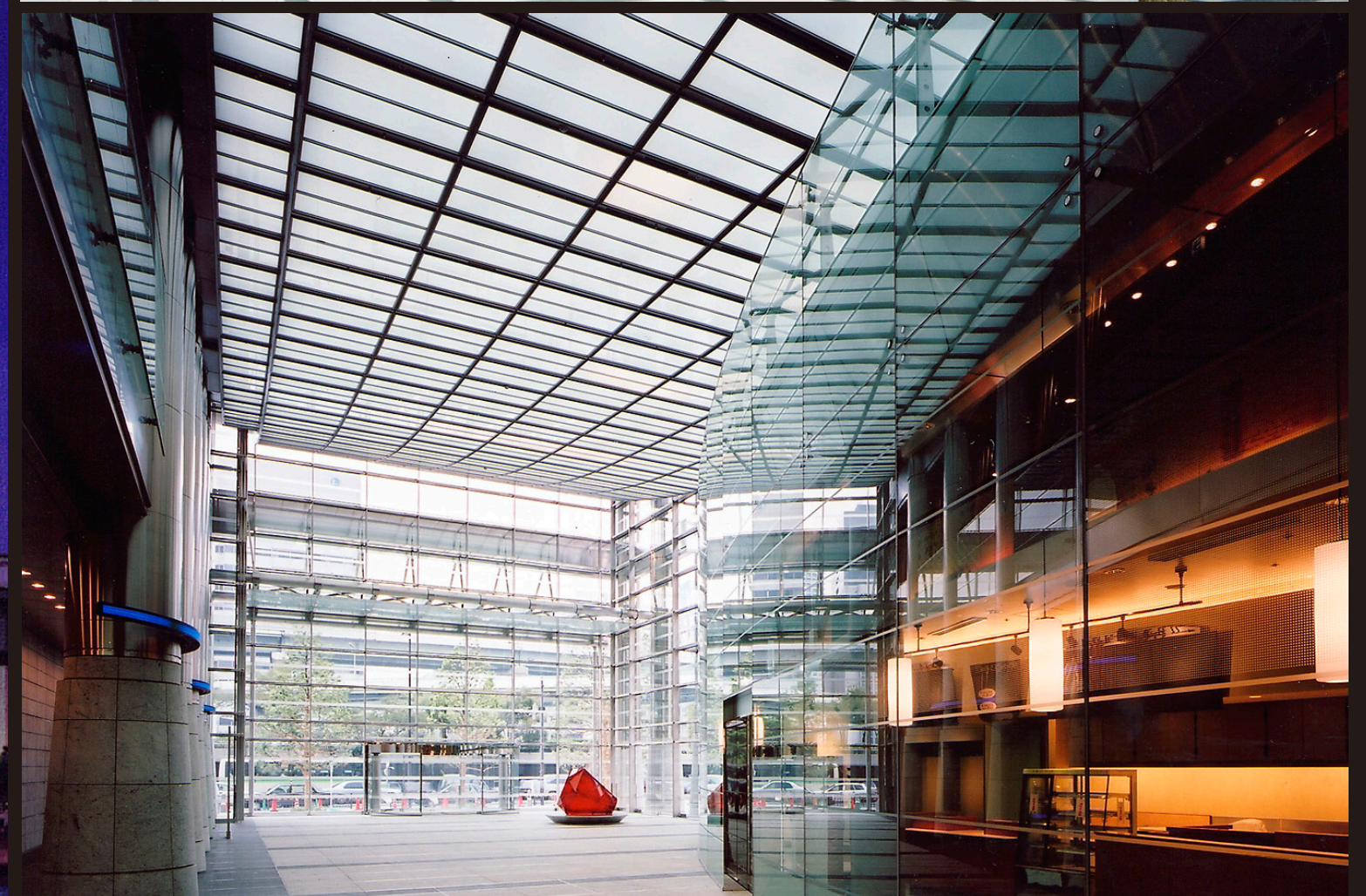
NAKANOSHIMA MITSUI BUILDING, OSAKA
