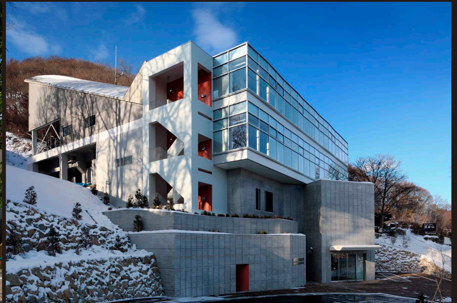
Mt. MOIWA ROPEWAY FACILITIES, SAPPORO
