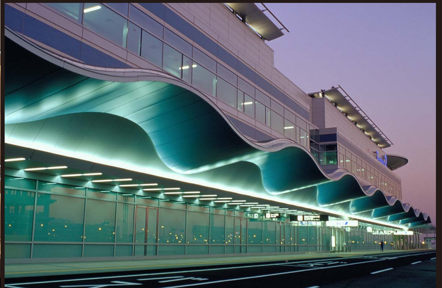
TOKYO INTERNATIONAL AIRPORT DOMESTIC PASSENGER TERMINAL2, TOKYO
